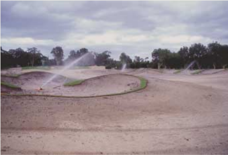
Bunker construction at the Bonnie Doon Golf Club in NSW
