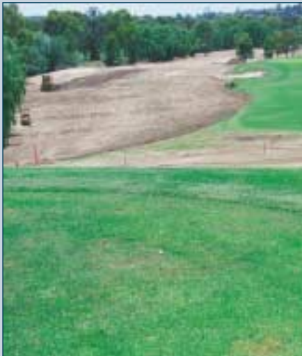
Construction of the new 1st at Freeway
