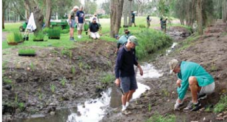
Mona Vale course staff and members during wetland system rehabilitation works
